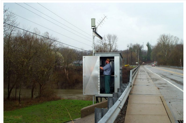
USGS hydrologic technician servicing streamgage 05599490 on Illinois Route 127 bridge across the Big Muddy River at Murphysboro, Illinois. Photo taken by Trent Legg, USGS, 03/22/2007.
